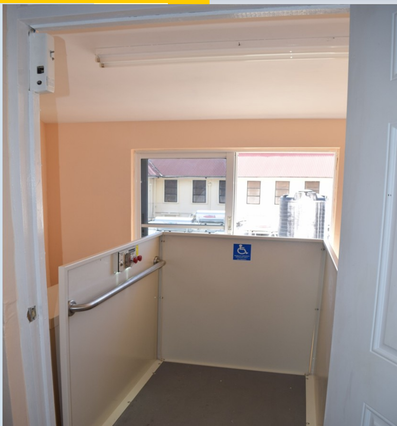
The newly installed wheelchair lift.
